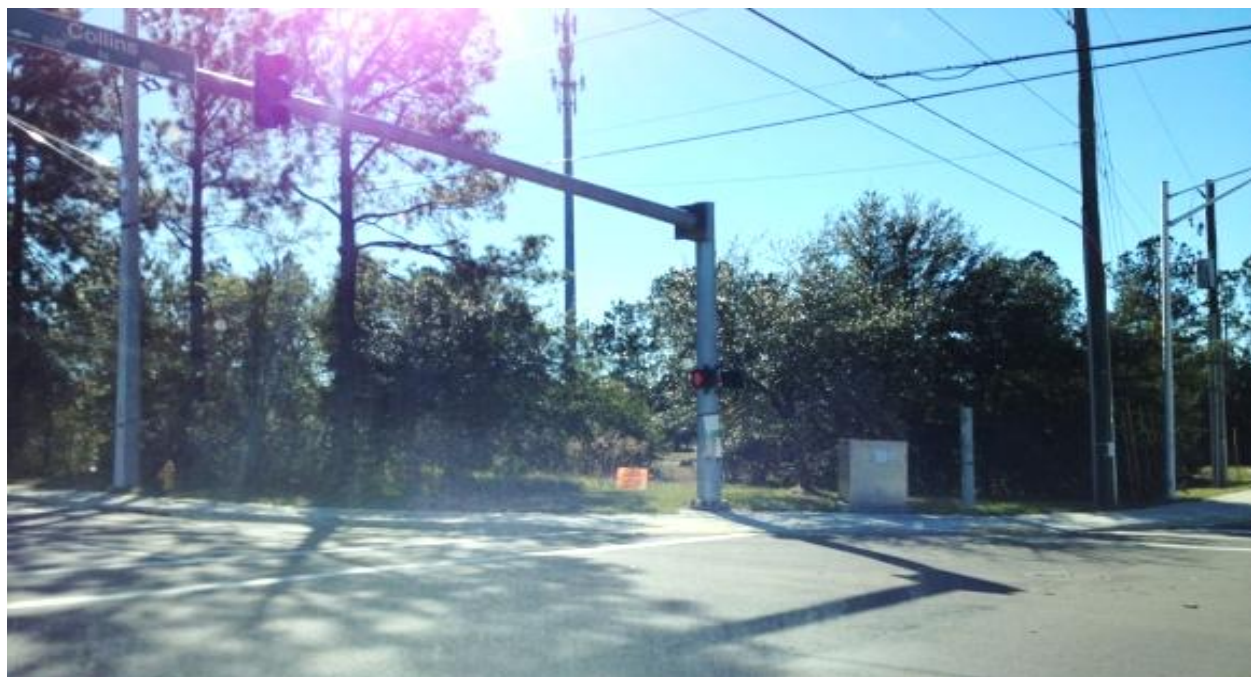
Facing southwest into the subject site from the Collins Rd./Shindler Dr. intersection
